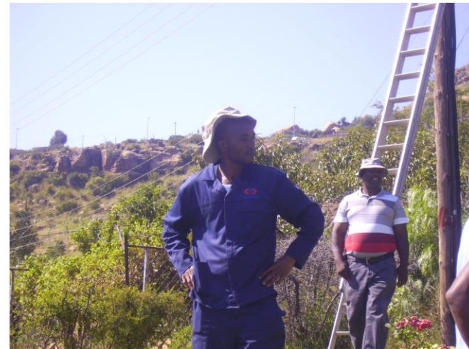
Figure 6: Grinpal Staff installing at Phuthaditjhaba
